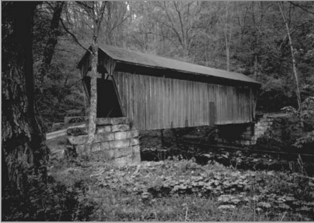
Fletcher Covered Bridge, Harrison County, W.Va. (IHTIA)
