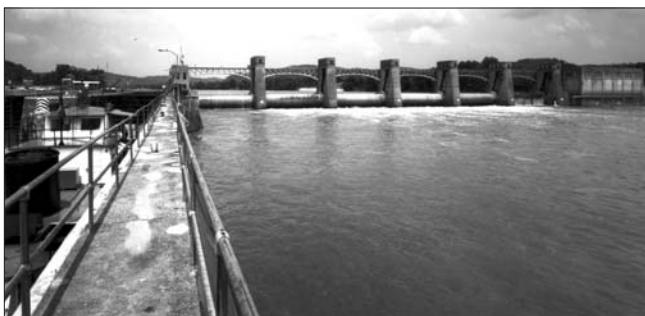
Top: Winfield dam under construction (U.S. Engineer Office, Huntington, W.Va., 1936); Bottom: Winfield Locks and Dam during expansion of locks. (John Nicely, ca. 1998)
