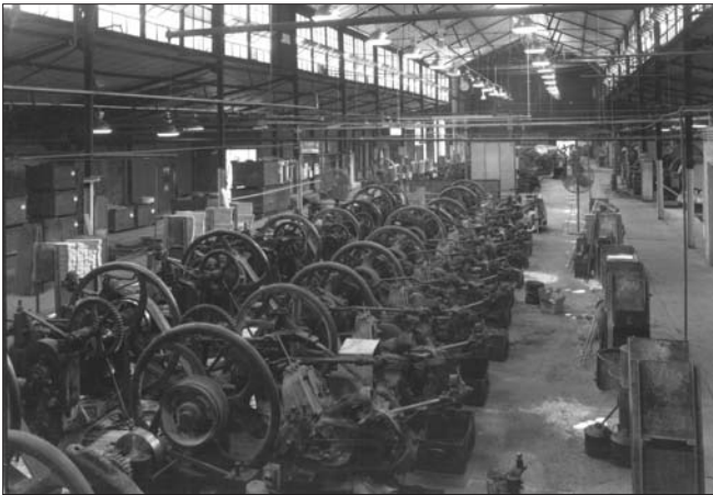
The Wheeling-La Belle Nail Company cut-nail plant was a stop on the Friday early bird tour. (Jack Boucher, 1990)
