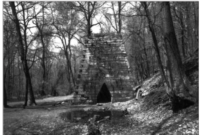
The 1836 Henry Clay Furnace, located at Coopers Rock State Forest, was a Sunday tour stop. (John Nicely, 1996)
