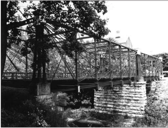
The twin spans of the of the Bollman Truss Bridge at Savage Maryland. In the background is the textile mill that the railroad spur served. (Michael Caplinger, 1999)
