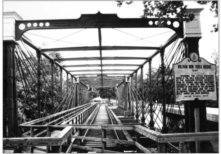
Looking north into the bridge portal. (Michael Caplinger, 1999)
